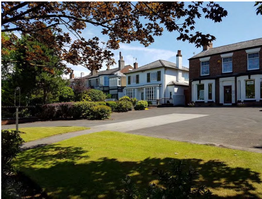
The early domestic character of Lord Street clearly remains in certain sections of the Conservation Area
