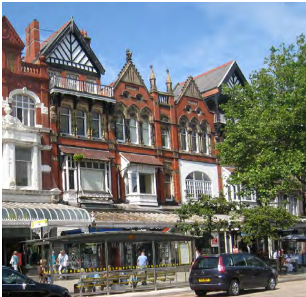
Albany Buildings. Note how the removal of the oriel window and rendering to the first floor, and the cutting back of the covered balcony on the third floor unbalances the symmetry of the building
