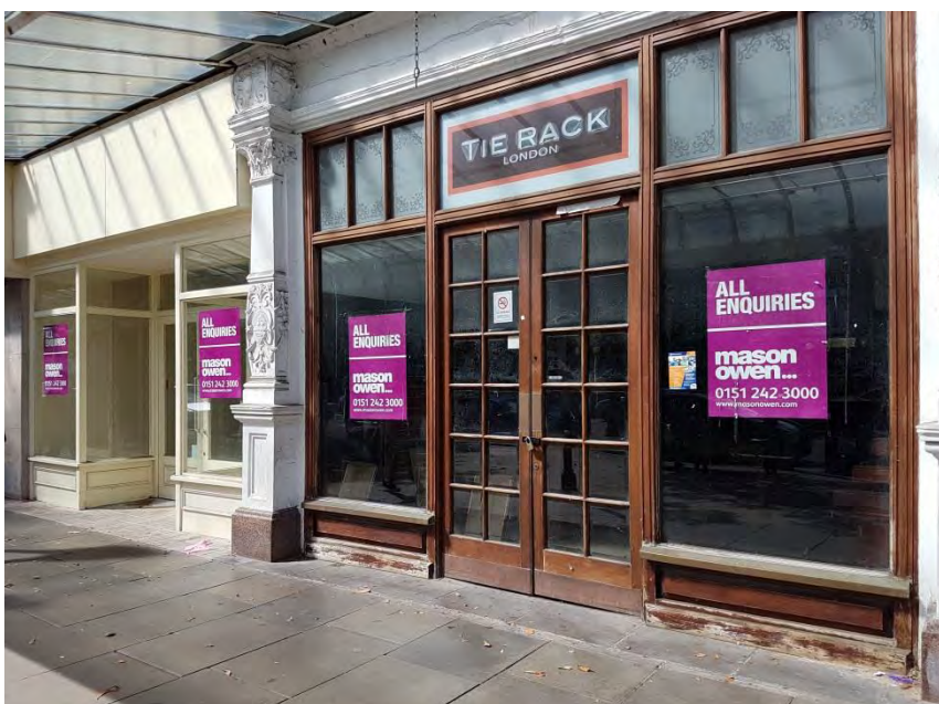
Where vacancy is obvious, the shopfront can appear lacking vibrancy and interest.
