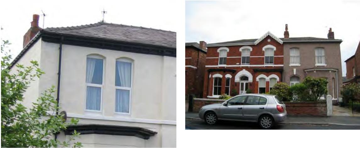
**Figure 28** Loss of detail and character owing to application of render
