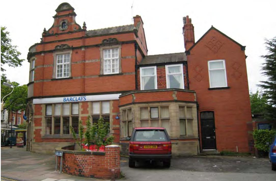
**Figure 43** The three casement windows on the lower section of the first floor have been altered from their original design. They would have been identical to the two original casement windows which still remain. The large panes are a much plainer and flatter solution; the lines of the window are less clean, with the opening section having narrower glazing
