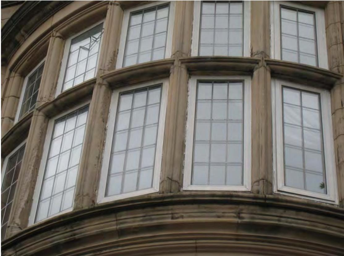
**Figure 44** The leadwork was originally much more elaborately designed. Note also the peeling-off decoration and the reflections
