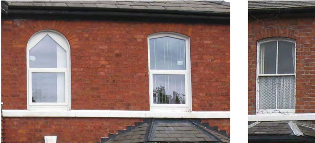
**Figure 52 Comparative photographs showing differences between traditional timber sashes and casement PVC replacements**
