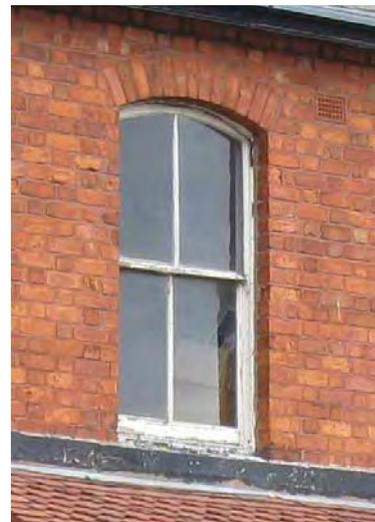
**Figure 30** Segmental arched head sash window
