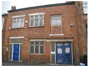
An example of poorly executed brick infills and structural amendments
