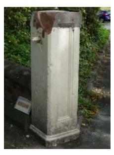
Photo 108: Damaged gate pier to Rosebank
