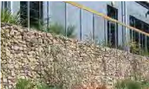
Swale Type 4 & 5- gabion bank on one side
