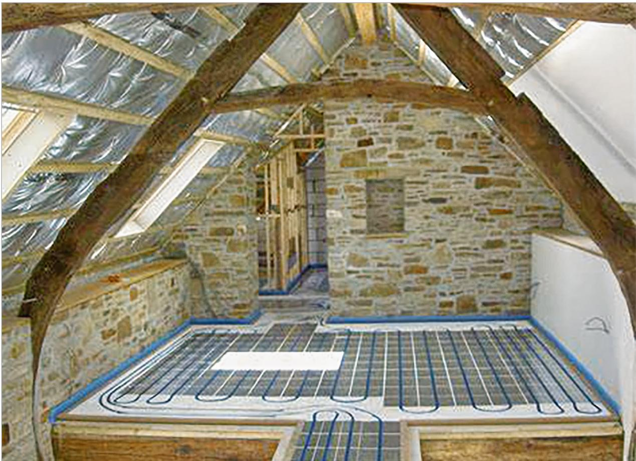
*If the floor can be lifted or historical flooring has been lost, then underfloor heating can be beneficial for evenly and consistently drying out solid floors in historic properties. This is an efficient way of maintaining your home.*
