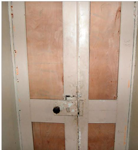
*Insulating panels that integrate with the original design and repairs to cracks do not harm the historic character of the door*
