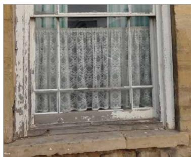
*Lost putty around glazing and a lack of repainting can lead to air leakages*
