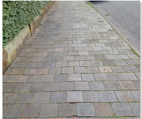
Natural wear and 'unevenness' that is part of the character of the Southport Paviers.
