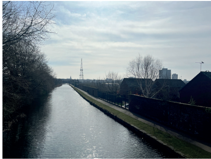
View from Linacre bridge looking south towards the gas works and telephone mast
