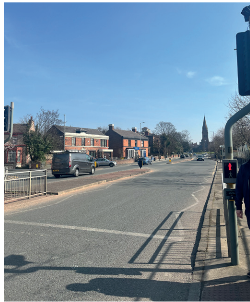
Pedestrian crossing on Merton Road to Bootle Village. The mansion house typology can be seen here. Christ Church at the top of Merton road in the background.
