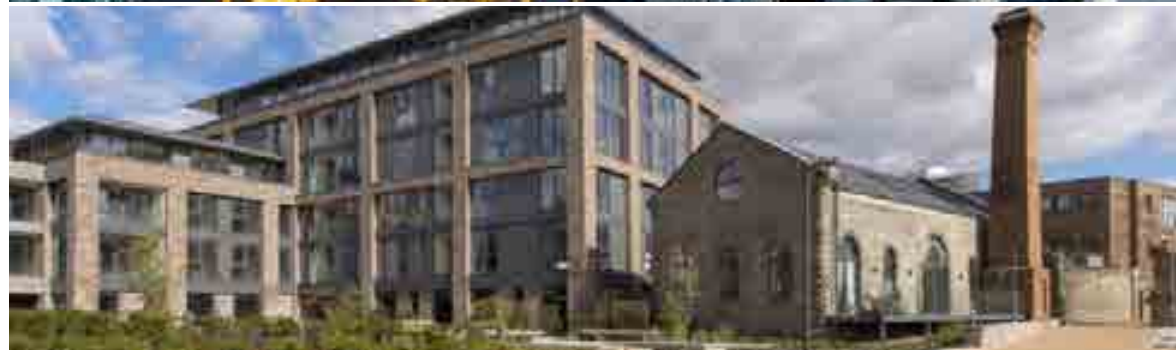
Right: Examples of waterside regeneration using a mix of new build and creative reuse can inform and inspire key principles and concepts and can help us to understand different design 'scenarios' that future development may encounter (Top: Brentford Lock, Bottom: Brandon Yard, Bristol) (Image credits: Canal and River Trust and XXXXXXX)
