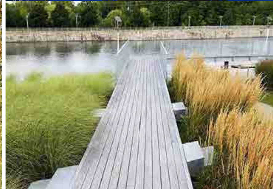
Far left: Canalside homes at Wichelstowe, blending an urban aesthetic with a green canal edge (image credit: David Wilson Homes)
