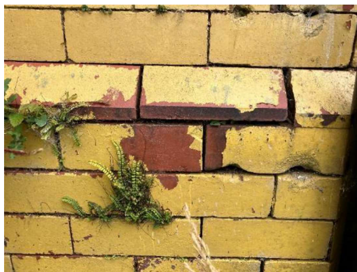
Figure 14: Decay of mortar joints (front elevation).
