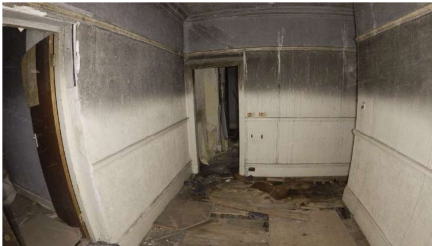
Figure 40: Fire / smoke damage noted to decorative linings of ground floor walls.
