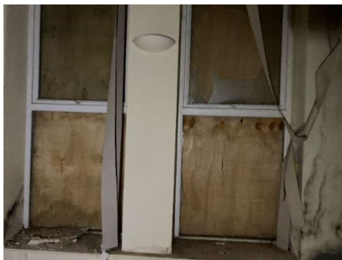
Figure 17: Failed glazing units to ground floor uPVC windows, Building 3.
