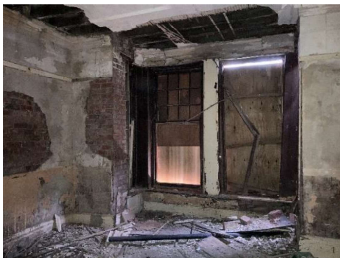
Figure 18: Severe deterioration of timber windows to Building 1, ground floor.
