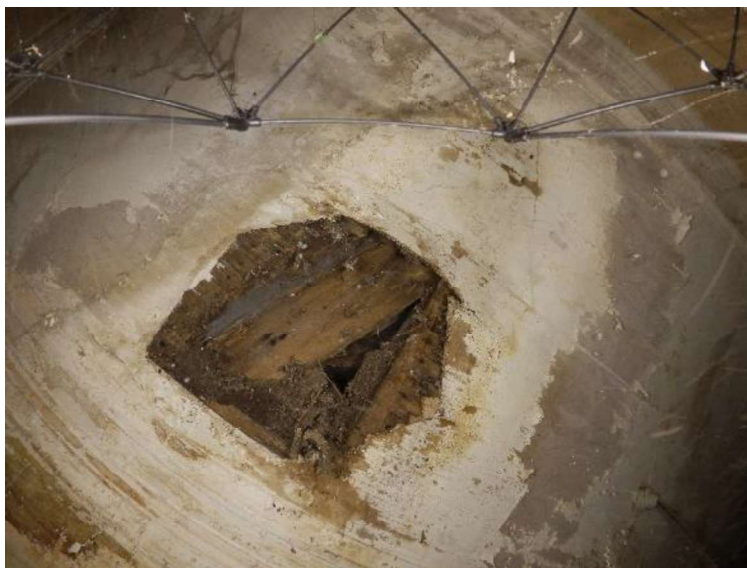
Figure 28: Slates exposed to underside of roof covering.
