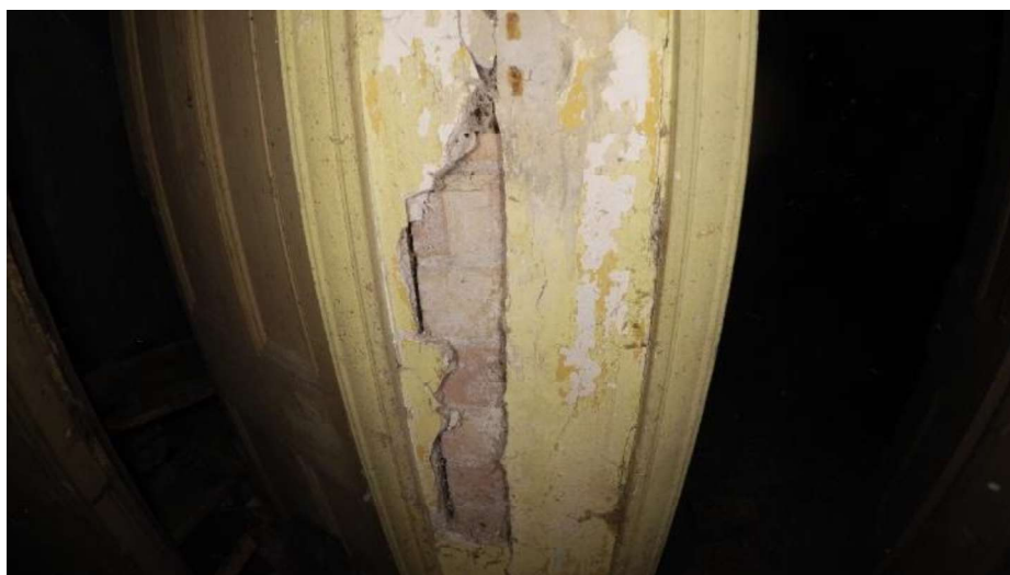
Figure 32: Deterioration of plasterwork to second floor.
