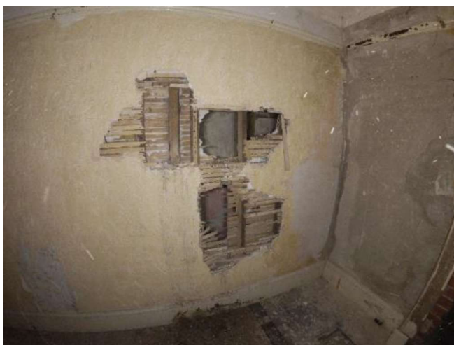
Figure 22: Partial collapse of lath and plaster partition to first floor.
