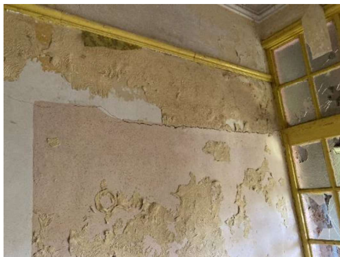
Figure 23: Horizontal cracking to ground floor wall.
