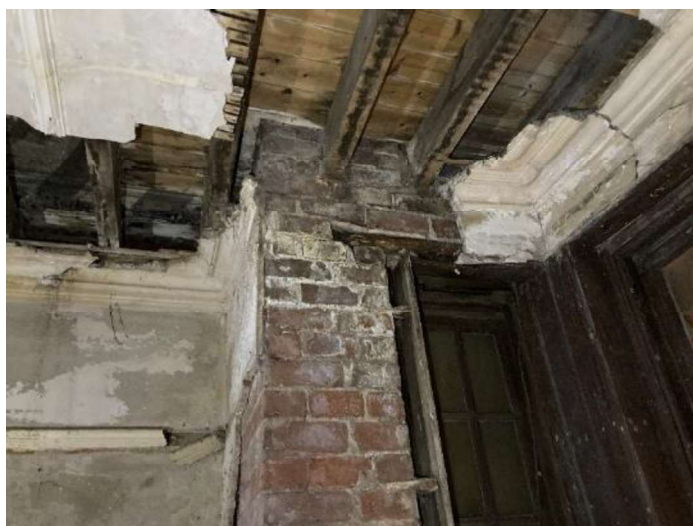
Figure 25: Failure of ground floor ceiling.
