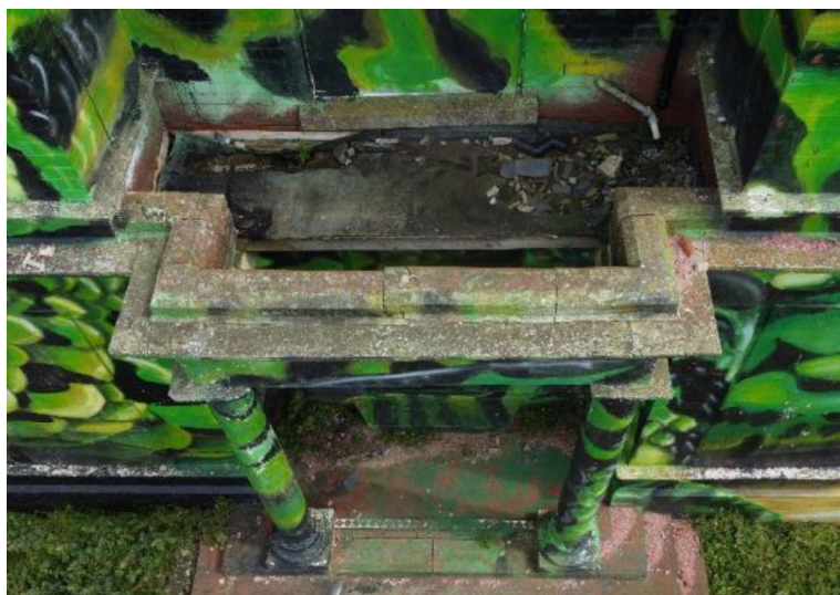
Figure 5: Failure of flat roof to entrance porch (front elevation).
