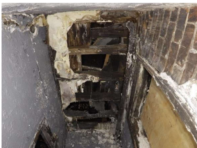
Figure 41: Fire damage to second floor timber floor structure.
