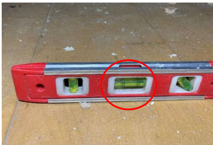
Figure 44: Spirit level showing sloping floors to ground floor.
