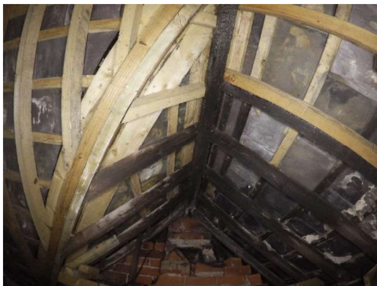
Figure 42: Fire damage to timber roof structure, and localised patch repairs.
