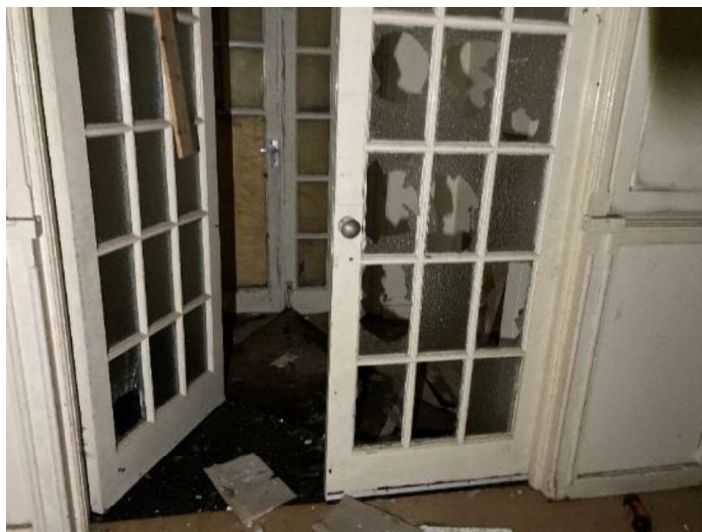
Figure 48: Failure of glazing panels to timber doors, Building 3, ground floor.
