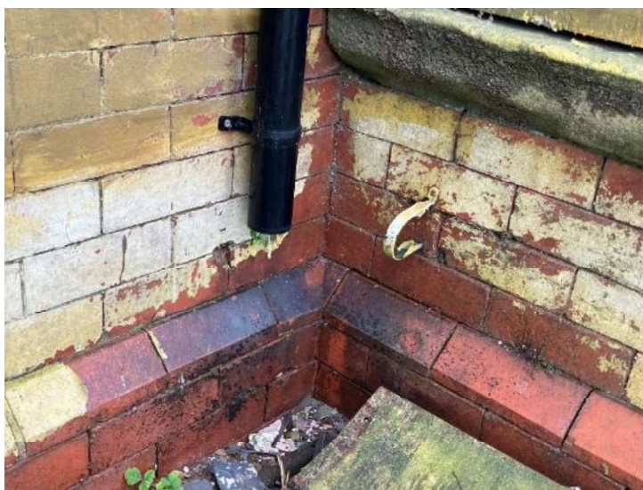
Figure 8: Lack of sufficient drainage system to downpipes.
