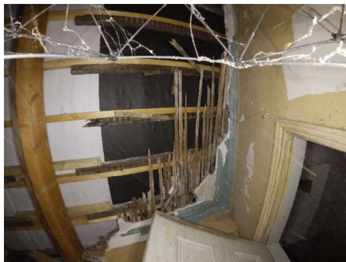
Figure 35: Patch repairs to natural slate roof covering visible from second floor ceiling.
