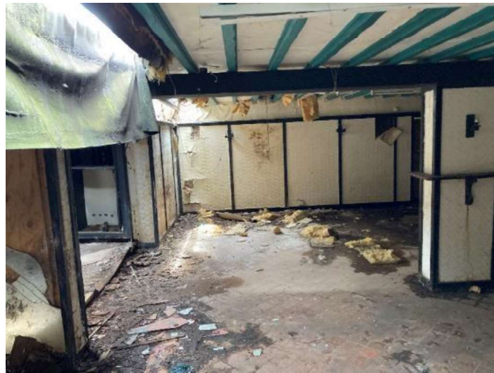
Figure 52: Stained / peeling decorative linings noted to walls.
