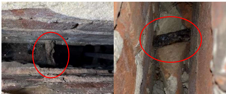
Figure 9: Corroded wall ties to cavity wall (front elevation).
