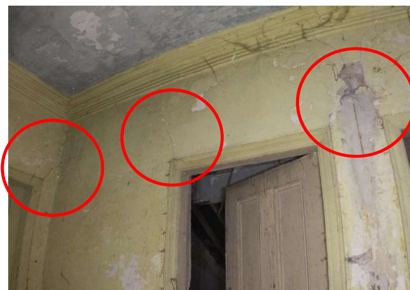
Figure 33: Cracking to plasterwork over openings on second floor.
