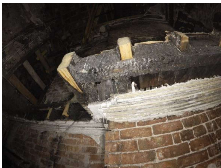
Figure 43: Fire damage to second floor timber floor structure, resulting in removal of timber joists.
