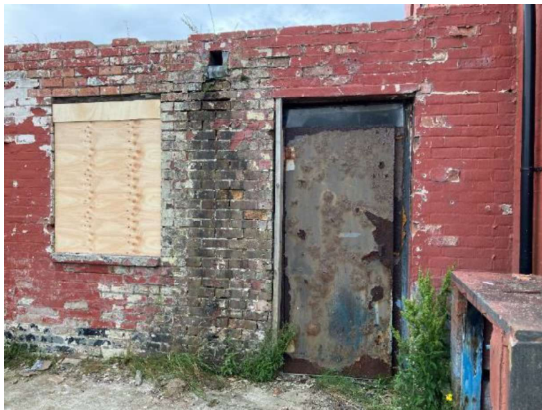
Figure 16: No downpipe installed to rear extension resulting in deterioration of brickwork.
