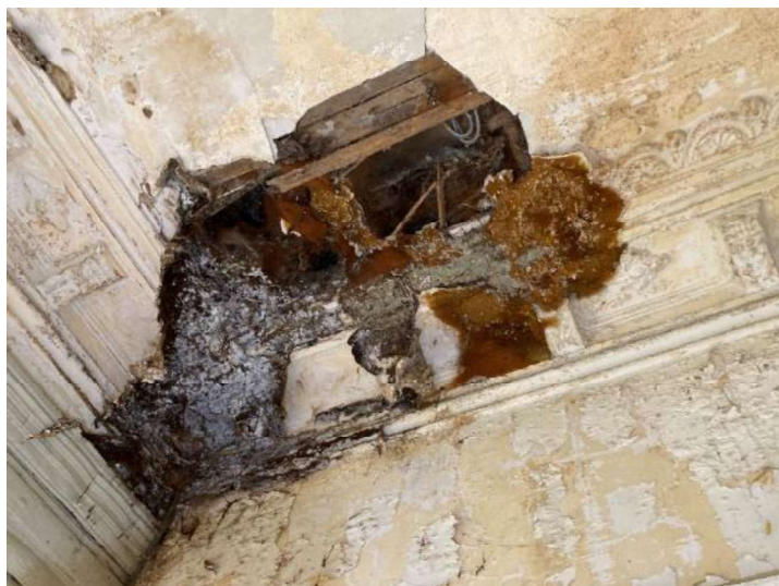
Figure 34: Dry rot noted to ground floor ceiling.
