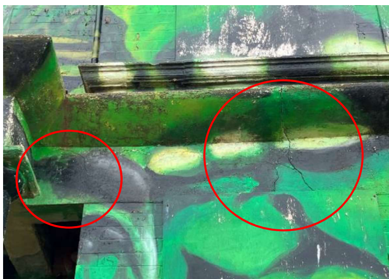
Figure 10: Cracking to stone sills (front elevation).
