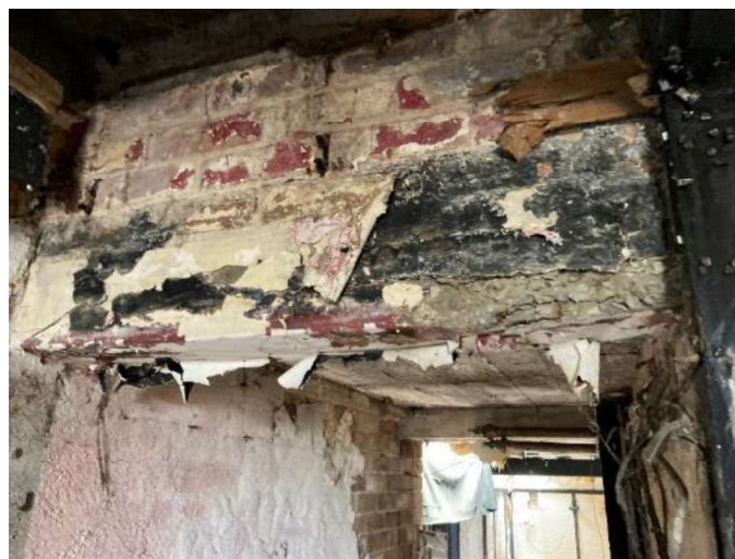
Figure 53: Failure of lintel.
