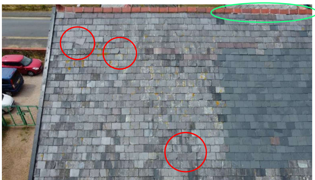
Figure 2: Aerial view showing condition of rear pitched roof.
