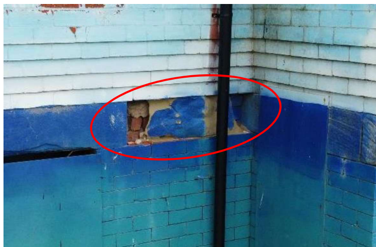
Figure 11: Erosion of stonework bank course to front elevation
