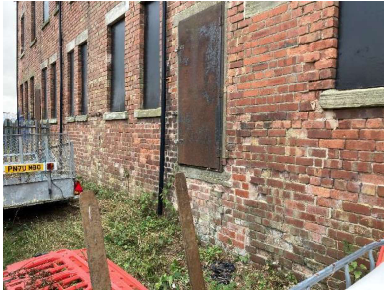
Figure 15: Spalling/cracking to brickwork and decay of mortar joints (rear elevation).
