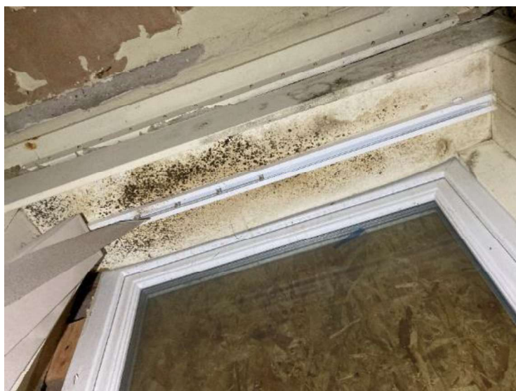
Figure 39: Black mould noted around ground floor window frames.
