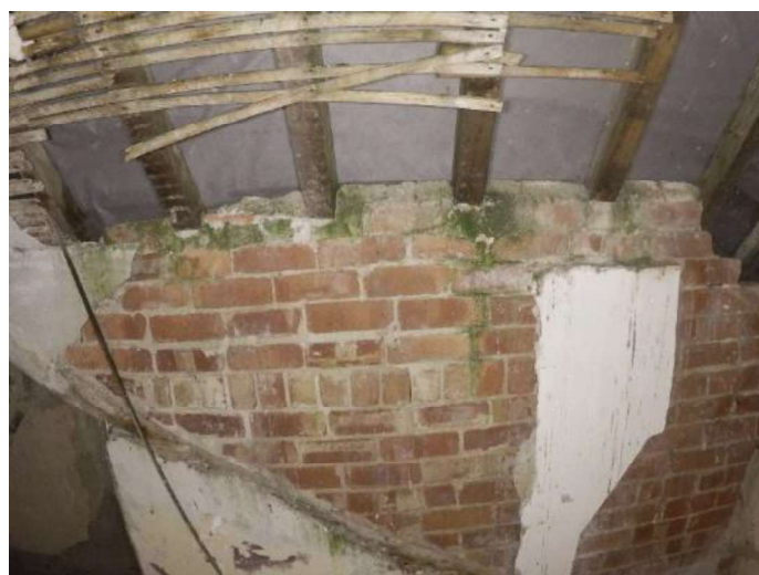
Figure 37: Penetrating damp to internal brickwork walls.
