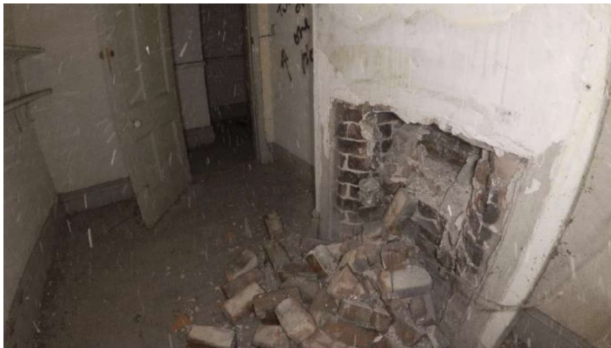
Figure 31: Partial collapse of brickwork chimney breast to first floor.
