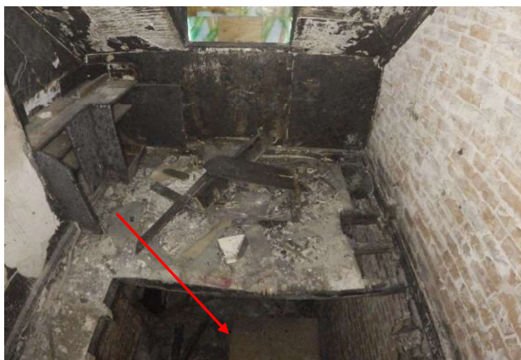
Figure 46: Fire damaged timber floor structure.
