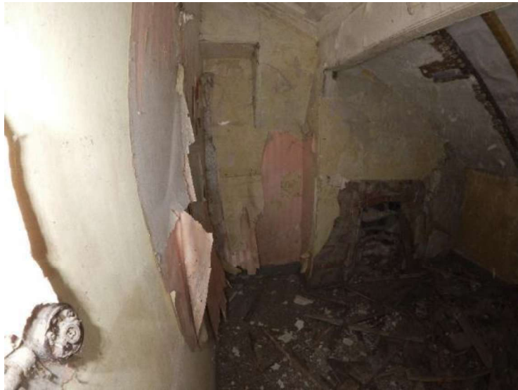
Figure 24: Deterioration of internal wall surfaces (second floor).
