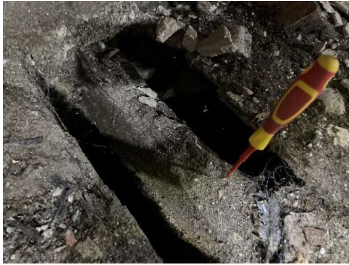
Figure 30: Timber decay to ground floor timber floor joists.
