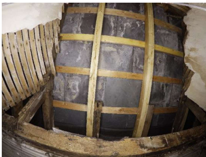
Figure 36: Original slate roof covering exposed to second floor.
