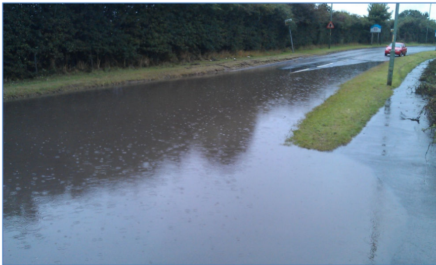
Figure 11: Bridges Lane, area A, taken 25/09/2012
